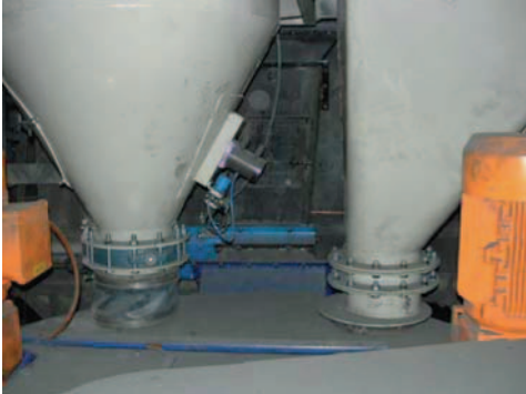
Loosening hard crusts with pneumatic linear vibrators
